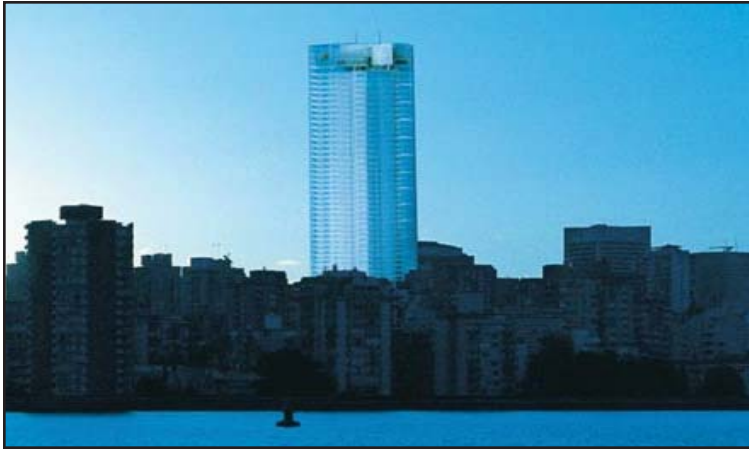
The new Shangri-La hotel, currently under construction illustrates the need to increase density in the Downtown core. How long can it be before strictly commercial office buildings are built to more than the current maximum 9 FSR?
