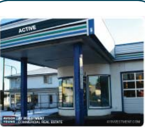
Corner Site Auto Service Station, Burnaby, BC
